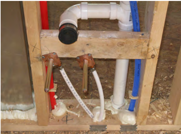
Plumbing penetrations between floors.
